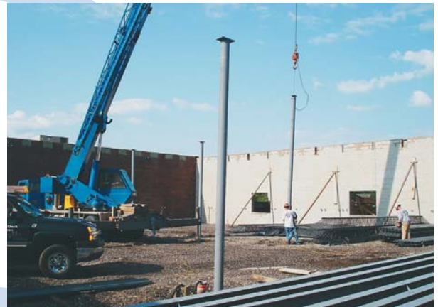
Ironworkers setting steel in August.
