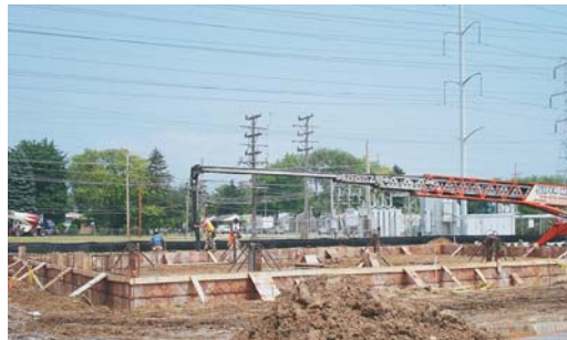
A concrete pump is used to pour the foundations.
